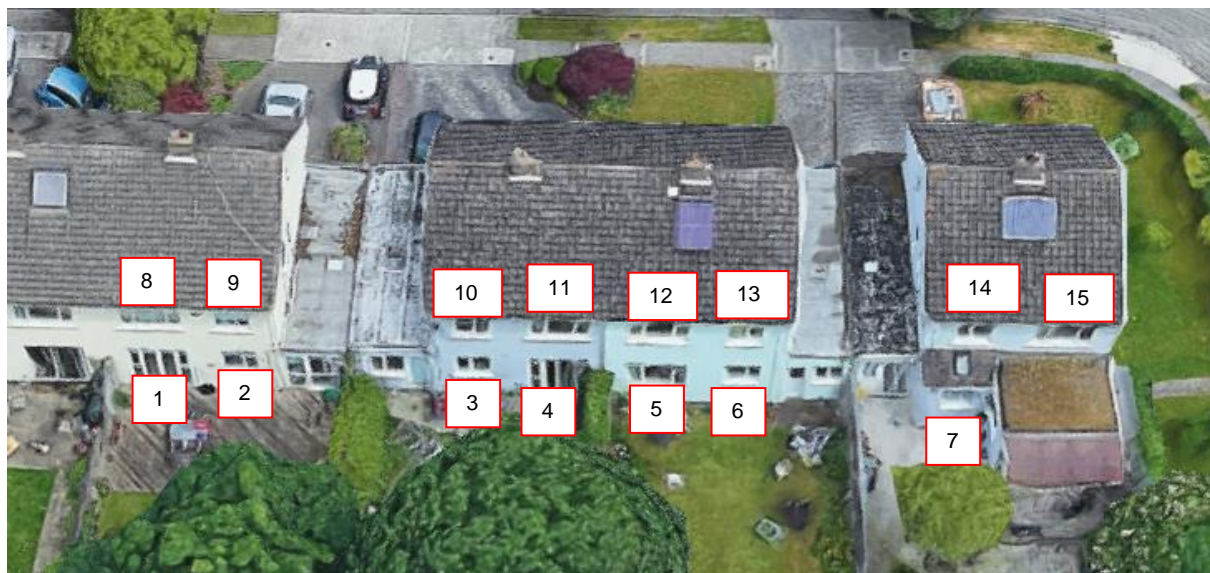
Figure 27 – Sensitive receptors at Lakelands CI (Source: Google Maps)
